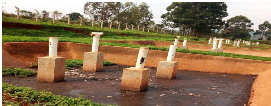
Figure 7: NTOBWE sewage sludge disposal site at GITEGA
