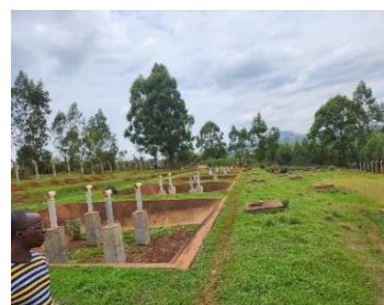
Figure : Waste sludge disposal unit
