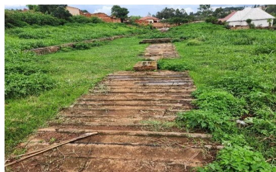
Figure 8 : Shatanya wastewater treatment plant
