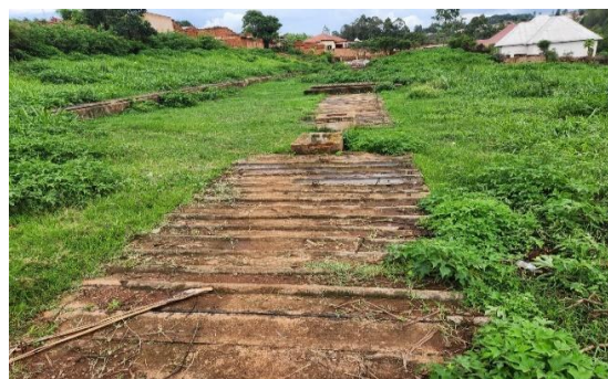
Figure 9: Station d'épuration Shatanya
